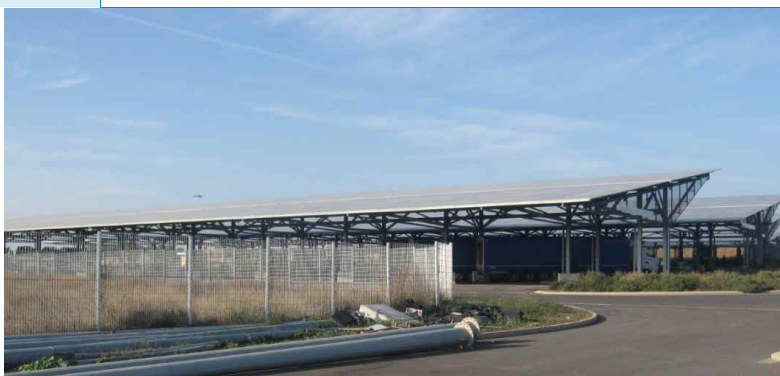
Figure 11 : Ombrières photovoltaïques (Via Europa) (Source : AMAE)
